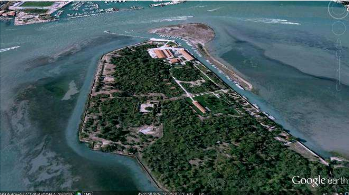
Vista verso ovest (Google Earth).
